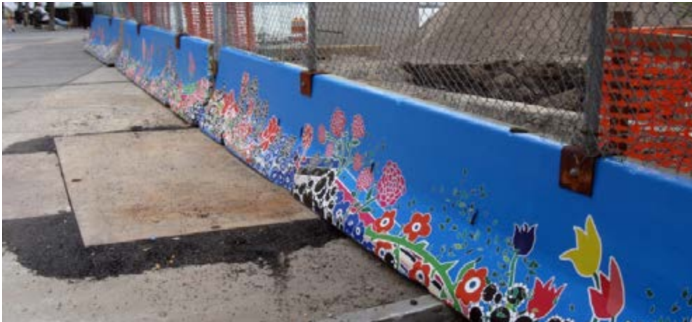
Installation View: Downtown Alliance BID , Construction Barriers
